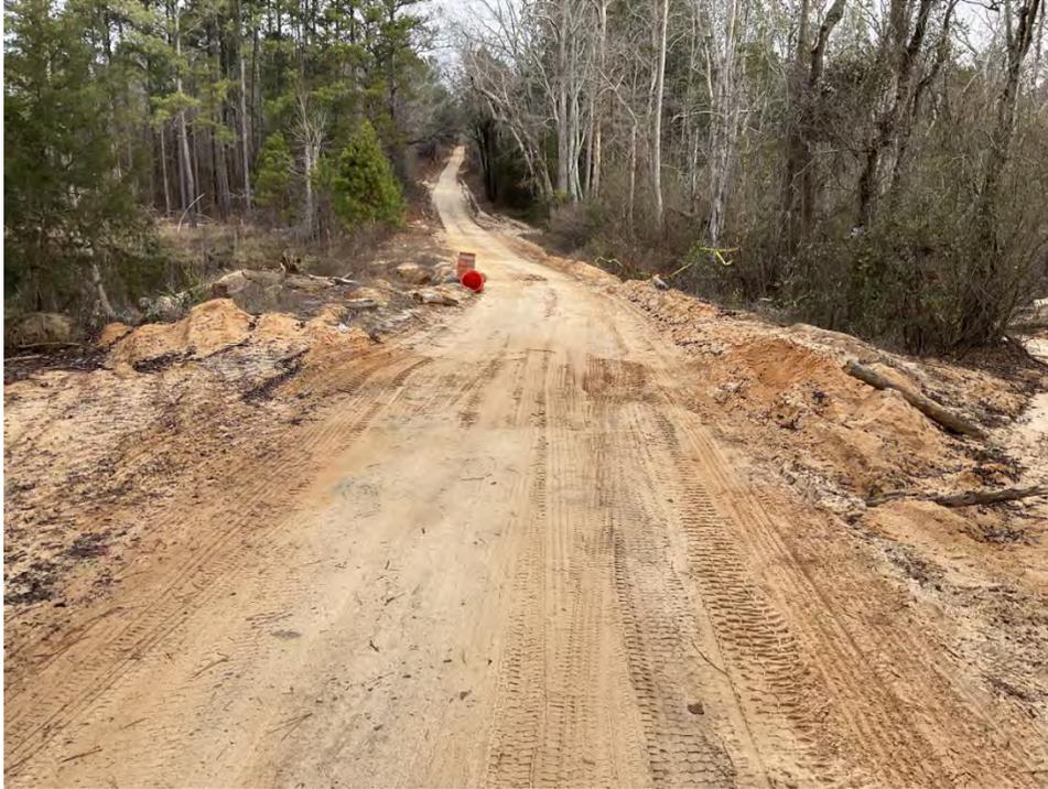
**Photograph 9.** Damaged road berm crossing Black Creek in archaeologically sensitive area along Volliedale Drive in SU 002. View north. Photographer: Adam Maskevich, Tetra Tech, January 13, 2022.
